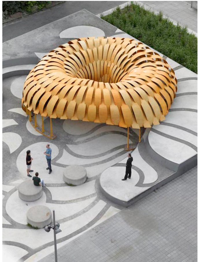
Images of Achim Menges' Bent wood structure and computer model. The systems are set up so that any bend in one corresponds to a bend in the other.
